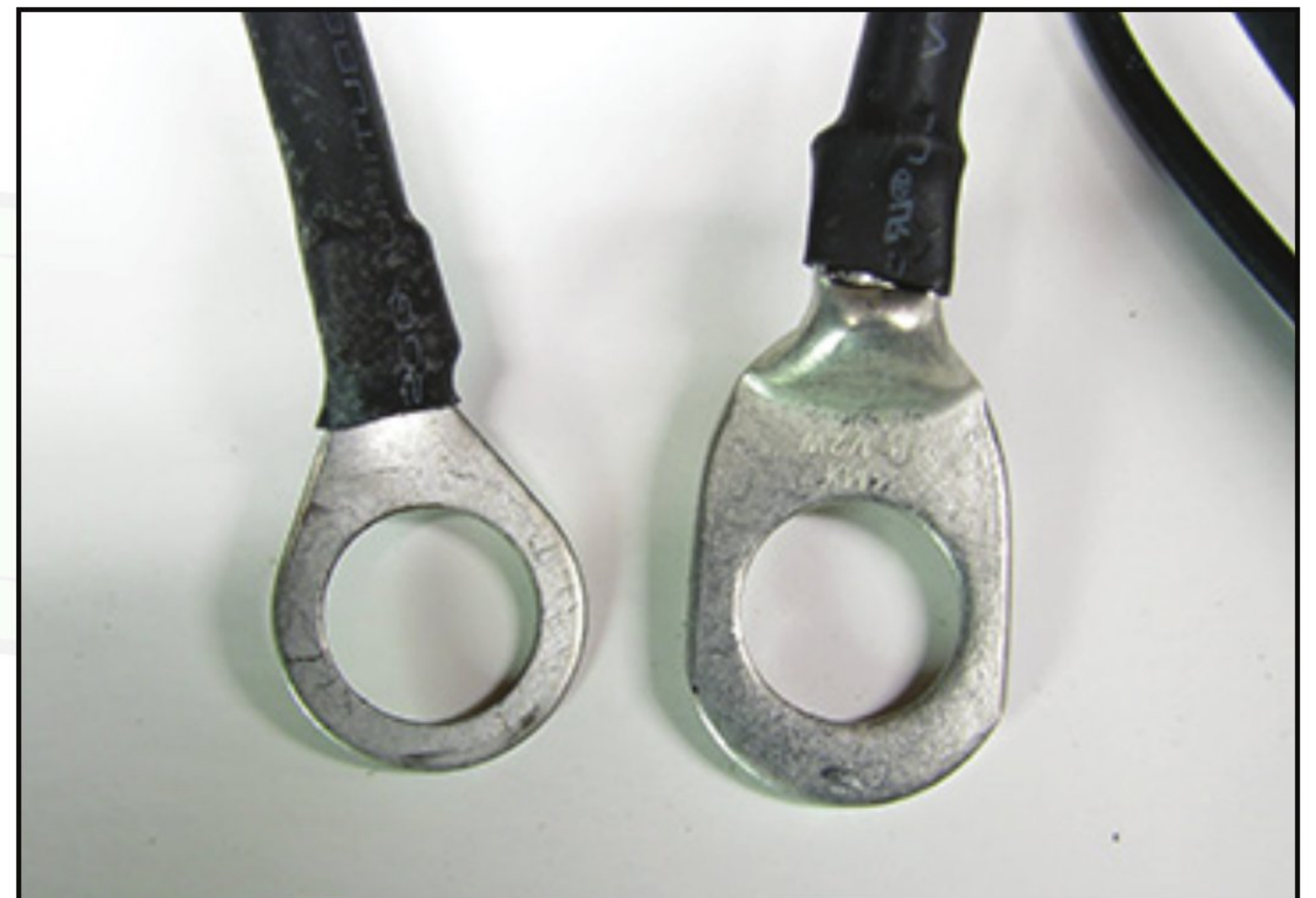
Figure 2 – Front view comparison of their B+ wire end terminals, Smart IMS (right) and original IMS (left).
