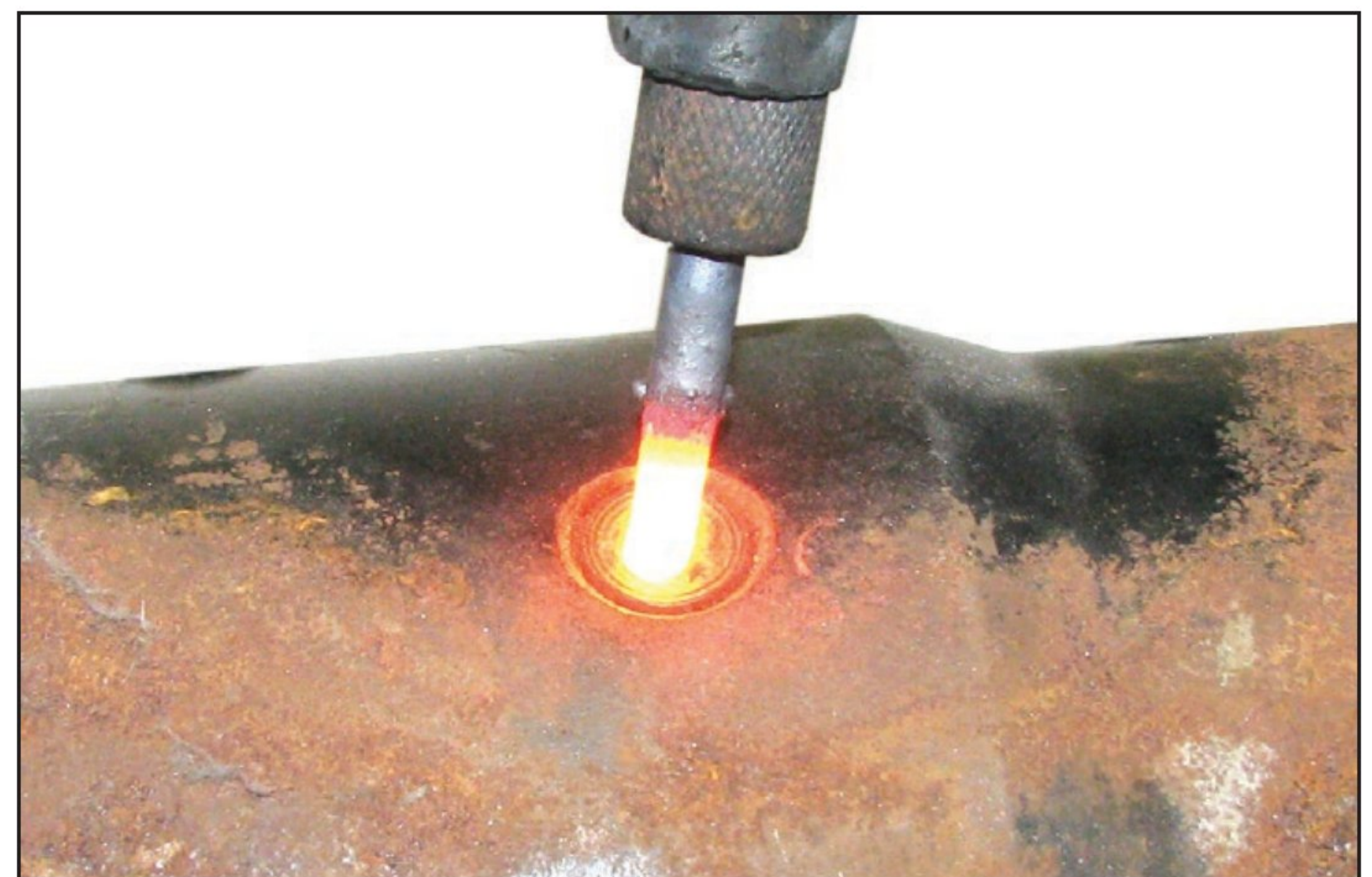
Figure 2—Heating with carbon rod.
