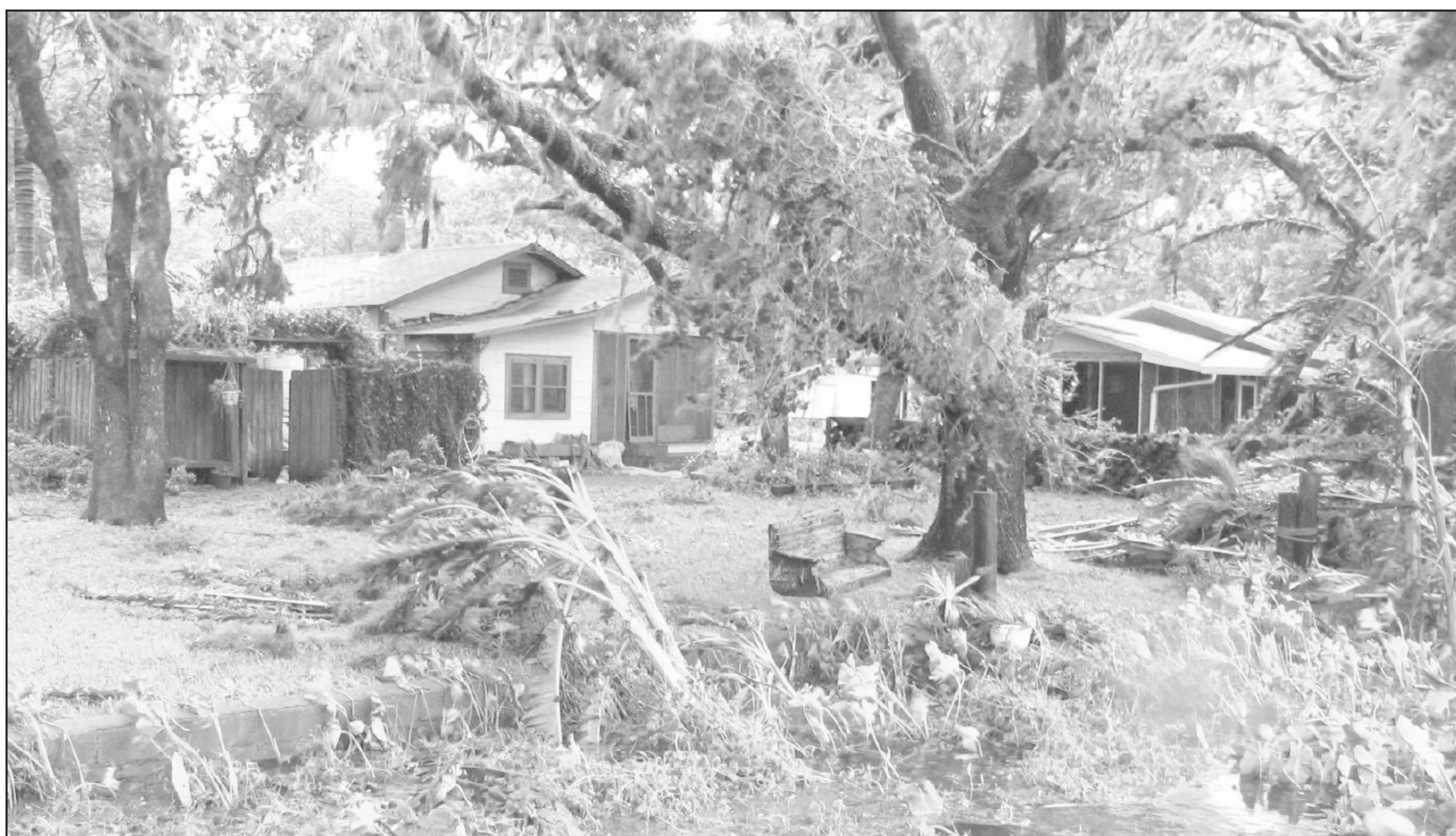
Residential damage was fairly substantial for Bob Thomas, owner of B&H Electric of Jacksonville.
