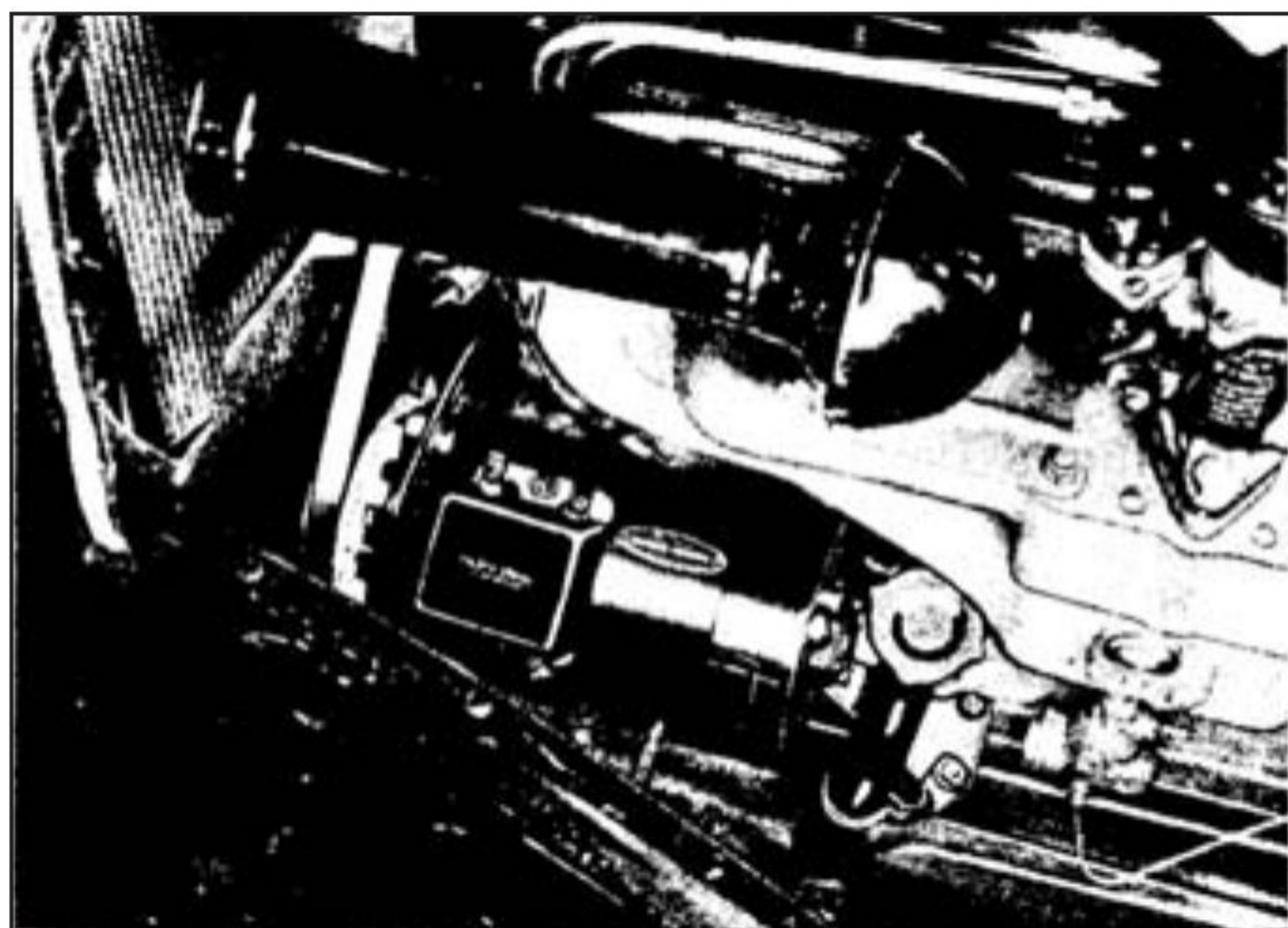
Figure 13—Installation of Class C generator with Step-voltage control mounted on generator
