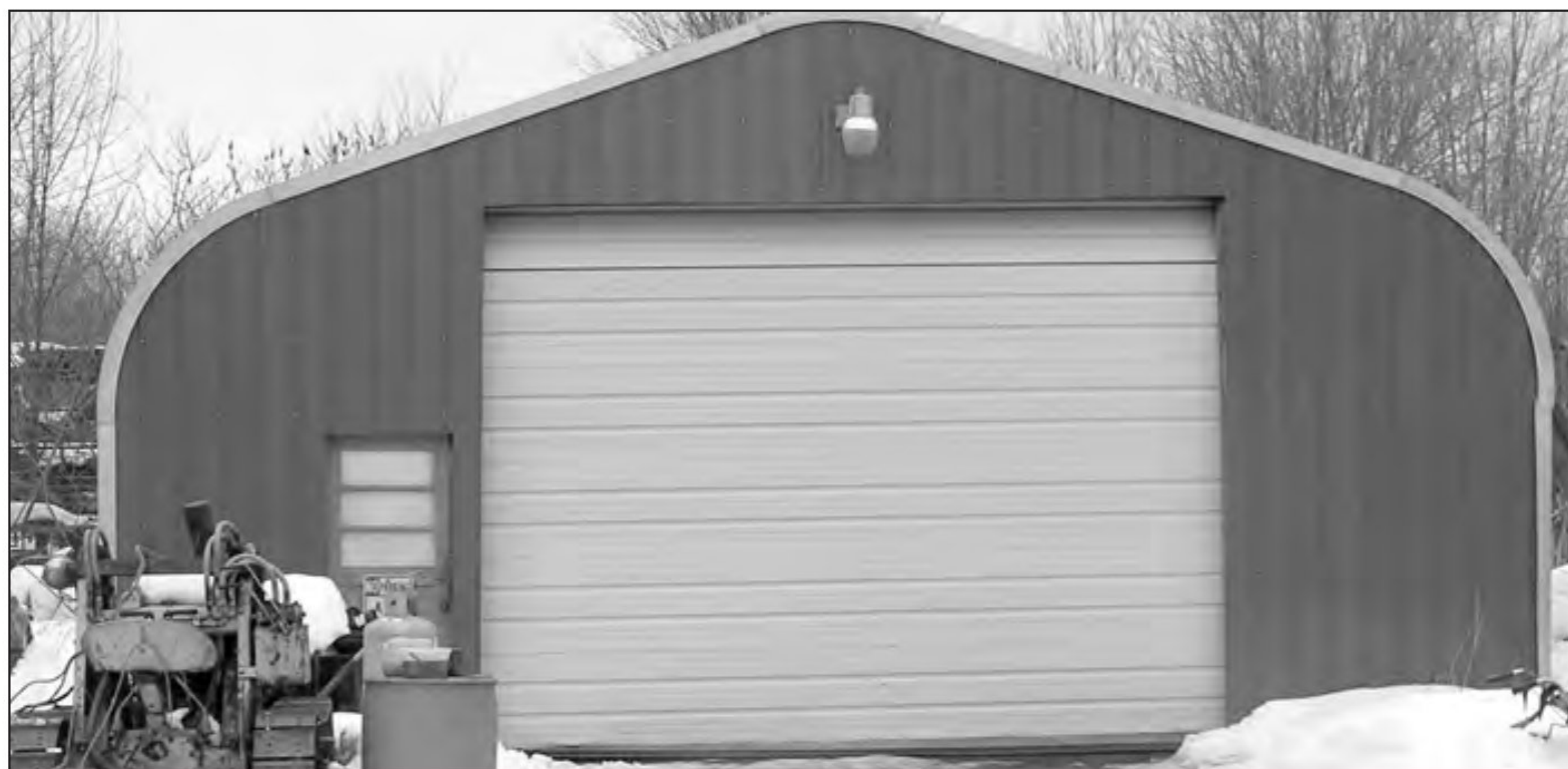
Gugino's Towing shop at their residence in North Collins, NY—simple, adequate and growing, in a rebuilding kind of way.
